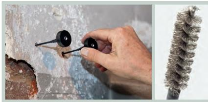
APPLICATION The brush electrodes are put into the pre-drilled hole
